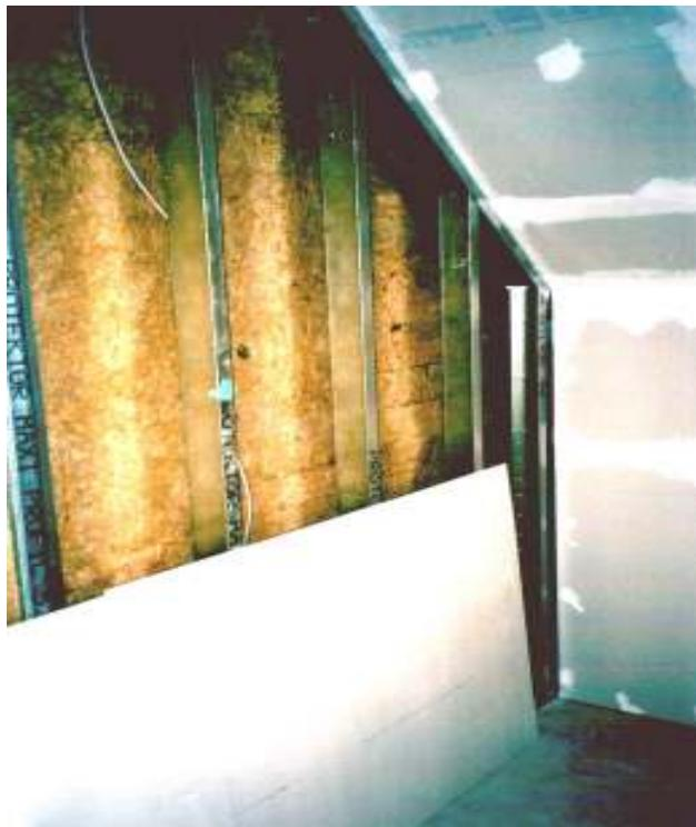
By grounding the metal trusses, you can reduce the electric alternating field to zero in all rooms concerned.
